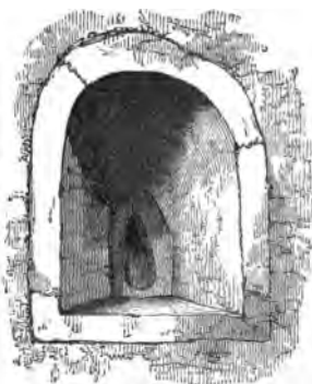
12. Window, Caversfield, Buckinghamshire, With small opening and very wide splay.
